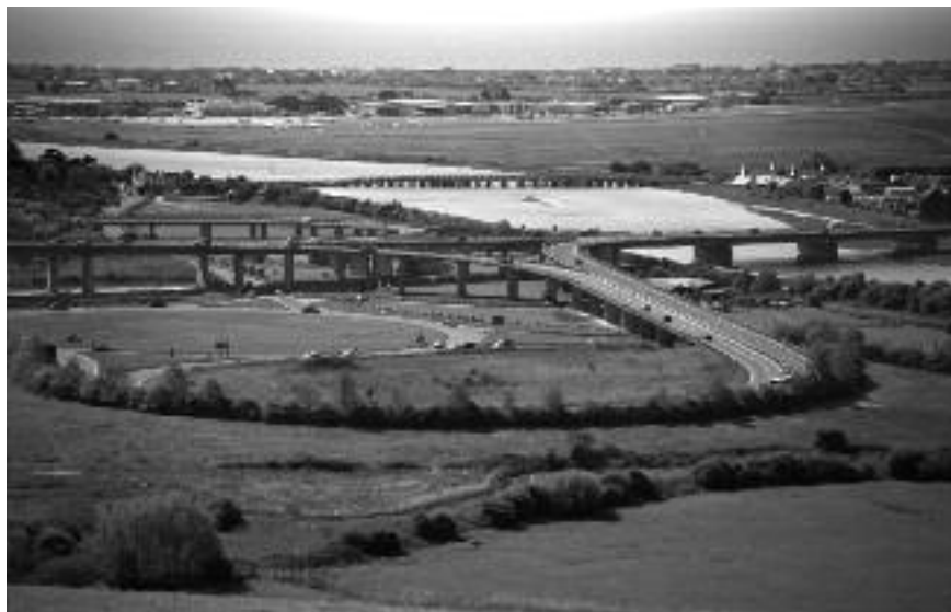
Two crossings of the River Adur: the enormous A27/A259 cloverleaf interchange dominates, compared to the original Old Shoreham Tollbridge in the background
